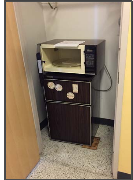
Microwave inside closet with a smoke detector- an unapproved location for Microwave use at WCM.
